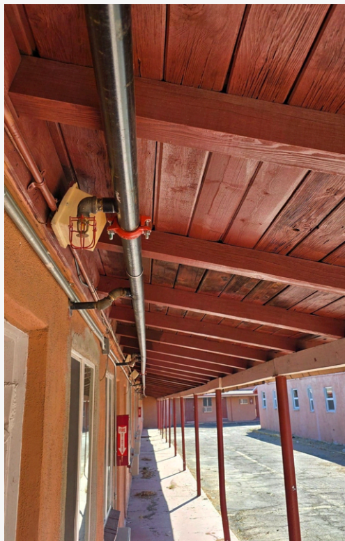
Sprinkler system installed
